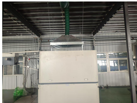
热熔胶贴标工位上方集气罩+软帘
